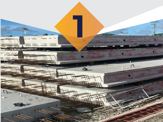
Prestressed Concrete Slabs
