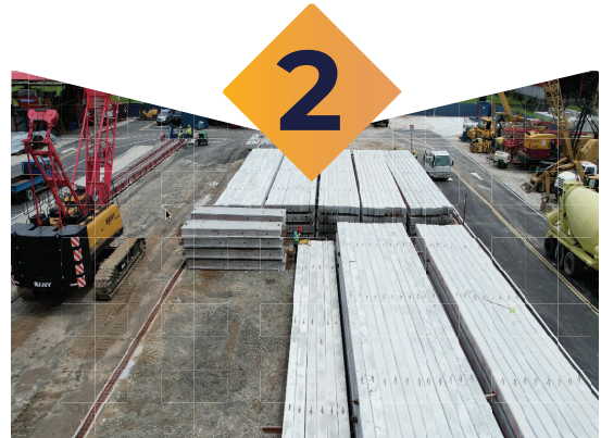
Prestressed Concrete Piles
